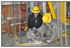
BM2 Eileen Pasion, with the assistance of BM2 Cheyenne Moscoso, verifies the lashings on this valve are properly torqued prior to lifting. (Photo by Sandy Hinz.)
