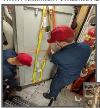
USS Stethem's DCFN William Nadler (left) and DC3 Nathan Harris position the balanced joiner door in preparation for installation. (Photo by LTJG Bryant
