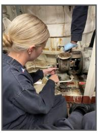
MM3 Shelby Hinnant prepares to remove a hot water recirculating pump casing in the restoration of a mechanical seal aboard USS Jason Dunham (DDG 109). (Photo by MMC(SW) Gordon Reichert.)
